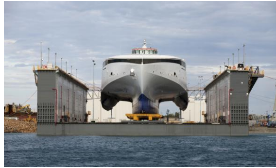
圖 2.2 Australian Marine Complex Floating Dock, http://www.ejelectrical.com.au/project-floatingdock.html
